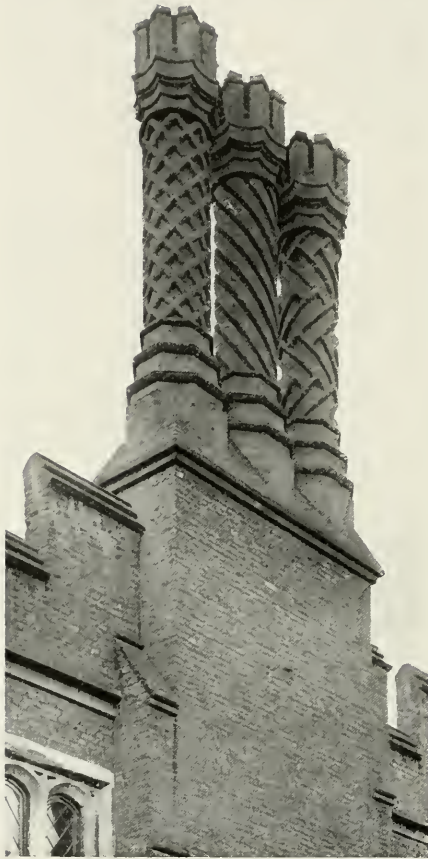
111. Chimney-stacks, Hampton Court.
